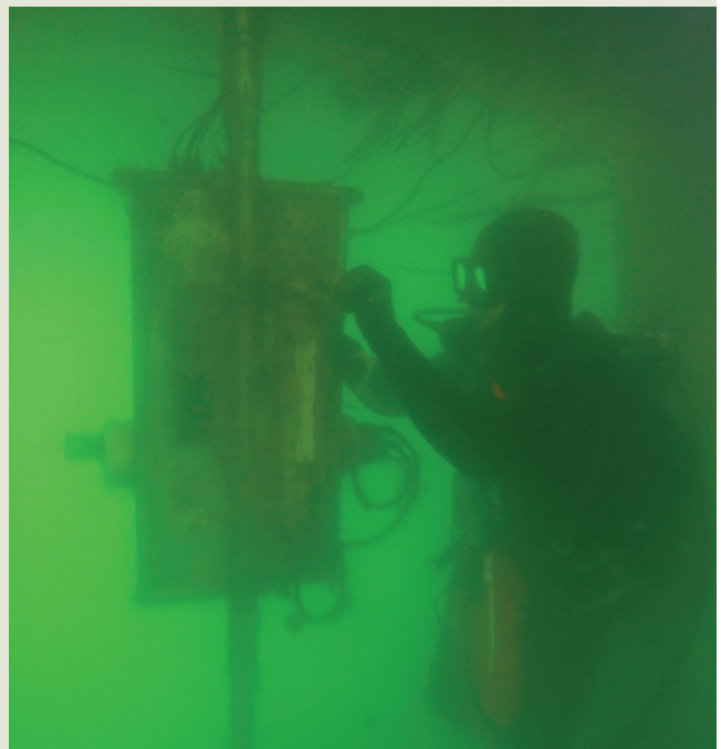
Senior Research Scientist Ian Robbins conducted maintenance on a monitoring sensor station at the north T-pier that measures water quality parameters such as temperature, pH, oxygen, and salinity. Photo courtesy of Dr. Ryan Walter.
