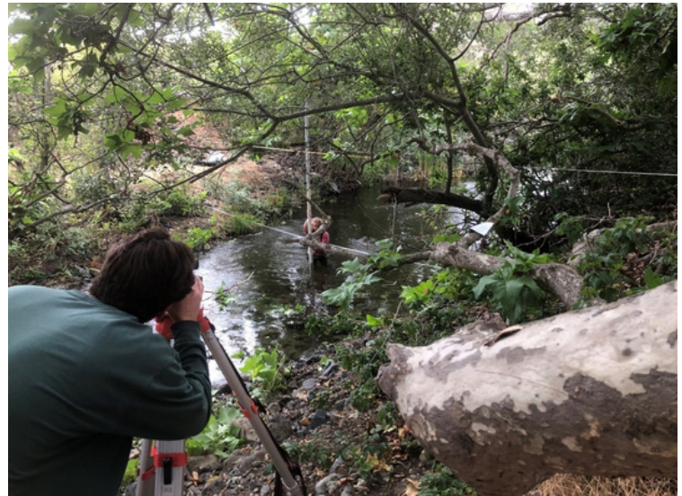
To survey a cross section, the team strings a measuring tape across the creek. A team member stands in the creek holding a stadia rod, which is like a large ruler. A second team member looks through an auto-level to read the numbers on the stadia rod. They collect these elevation measurements of the streambed at one-foot intervals, and the data is used to construct a cross-sectional view of the creek channel.
