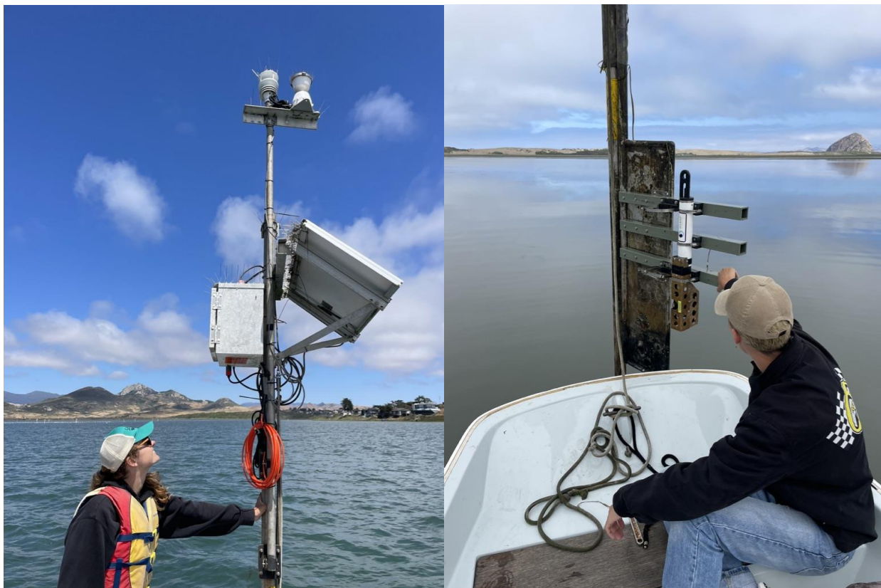
Figure 23. Cal Poly students check on the instruments at the back bay sensor station. The top of the station houses meteorological instruments for measuring weather parameters and a solar panel to power all the sensors (left). Water quality instruments are kept submerged but can be serviced by raising them above the water line with a pulley system (right). Photos courtesy of Ian Robbins.
