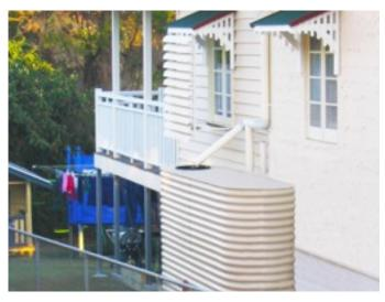
Rainwater from roof is stored in a *cistern* to be used for landscape irrigation.
